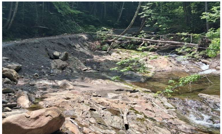
Figure 1. Washed out road and eroding stream bank with exposed bedrock and downed trees. Looking upstream on South Peacham Brook.
